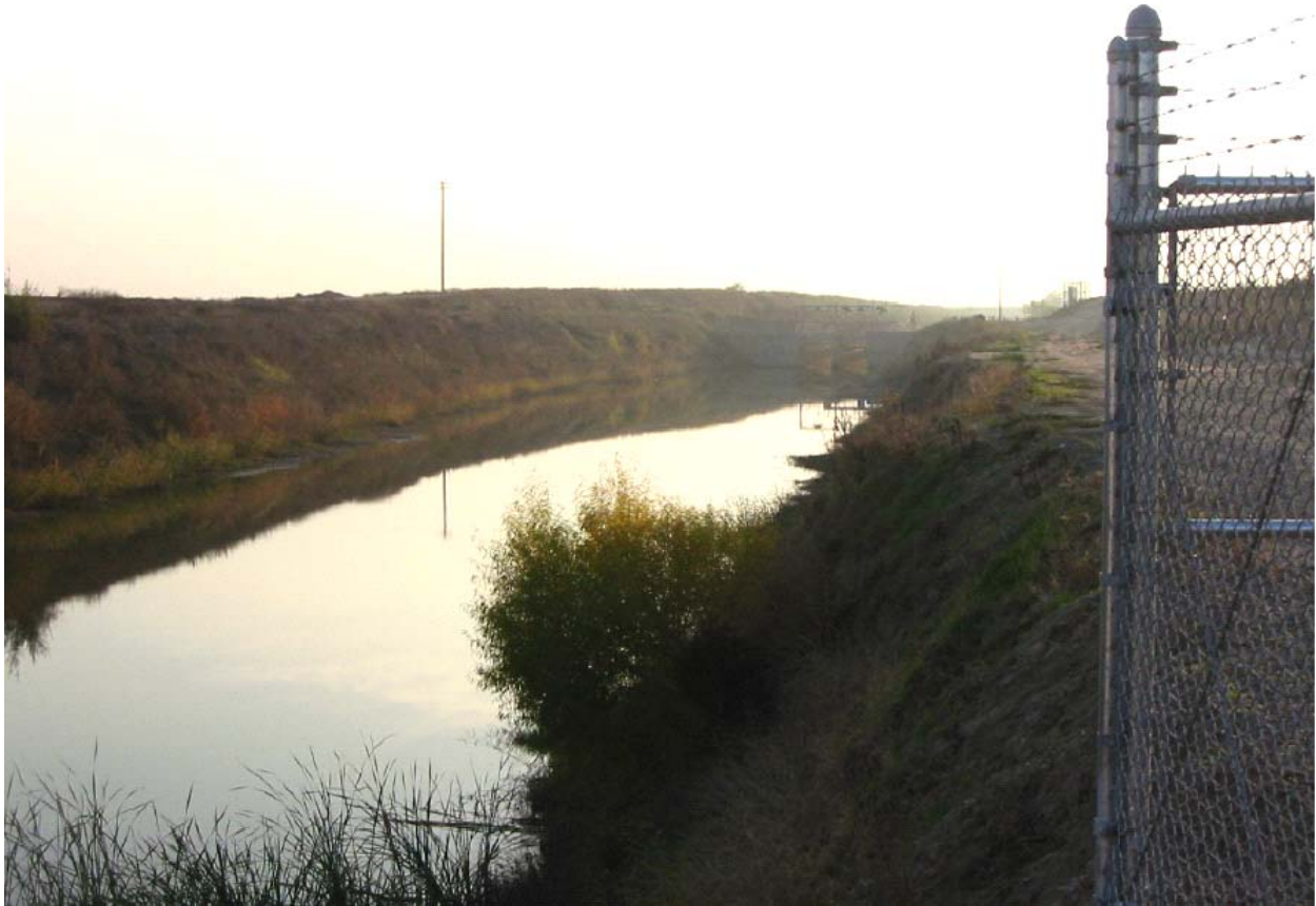
Figure J-3. Main intake canal showing first bank of lift pumps approximately 1/4 mile from the fish screen facility.
