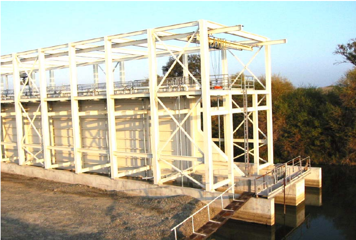
Figure J-2. Banta Carbona Irrigation District fish screen facility.
